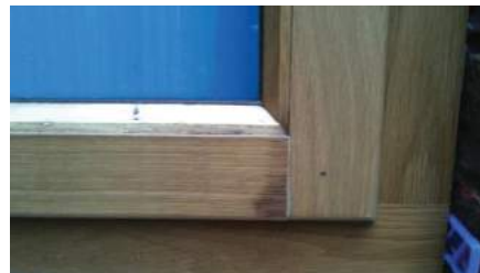
The natural movement of Oak can cause joints to open allowing water to enter, react with tannic acid in the timber causing characteristic staining
