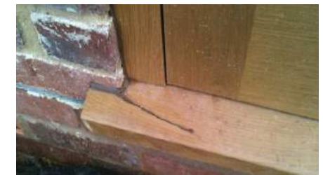
The surface of Oak joinery tends to split in service, disrupting the protective coating, allowing water to enter and react with tannic acid
